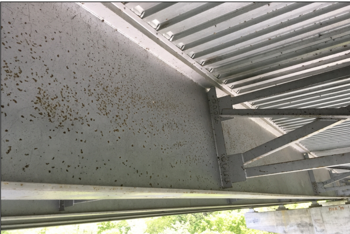
Paint condition in span #10. Worst case condition beam #3.
