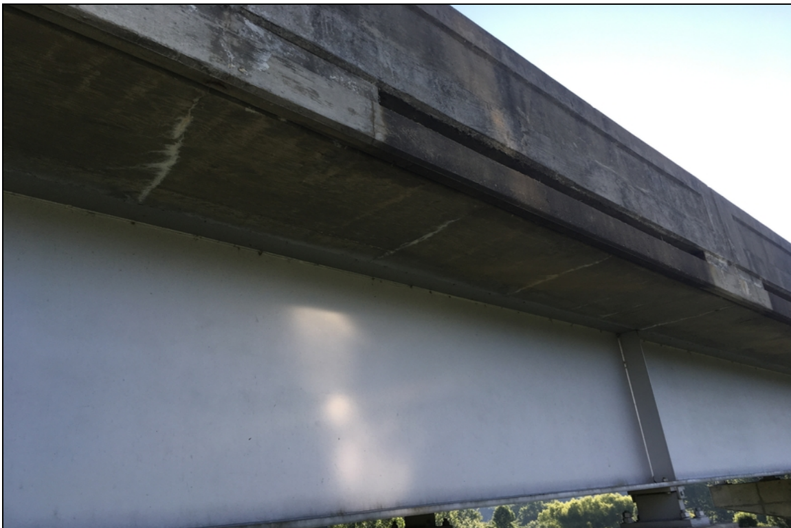
Efflorescence in the deck overhangs.
