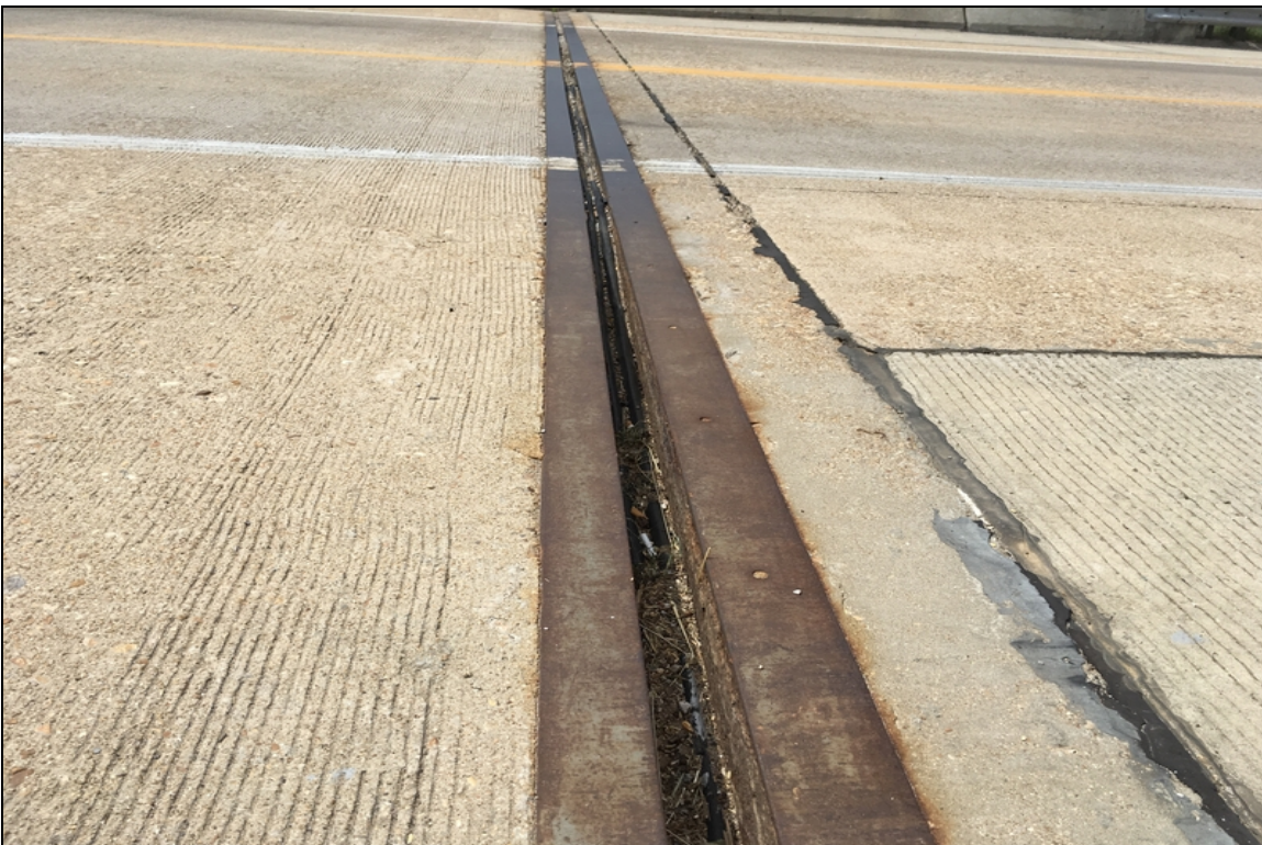
Condition of compression joint seal at abutment #1.
