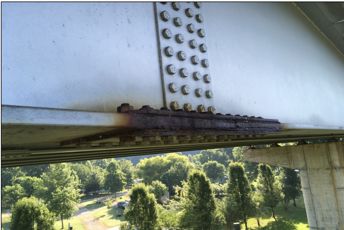
Splice panel corrosion on beam 6 in span 3 due to deck drainage.
