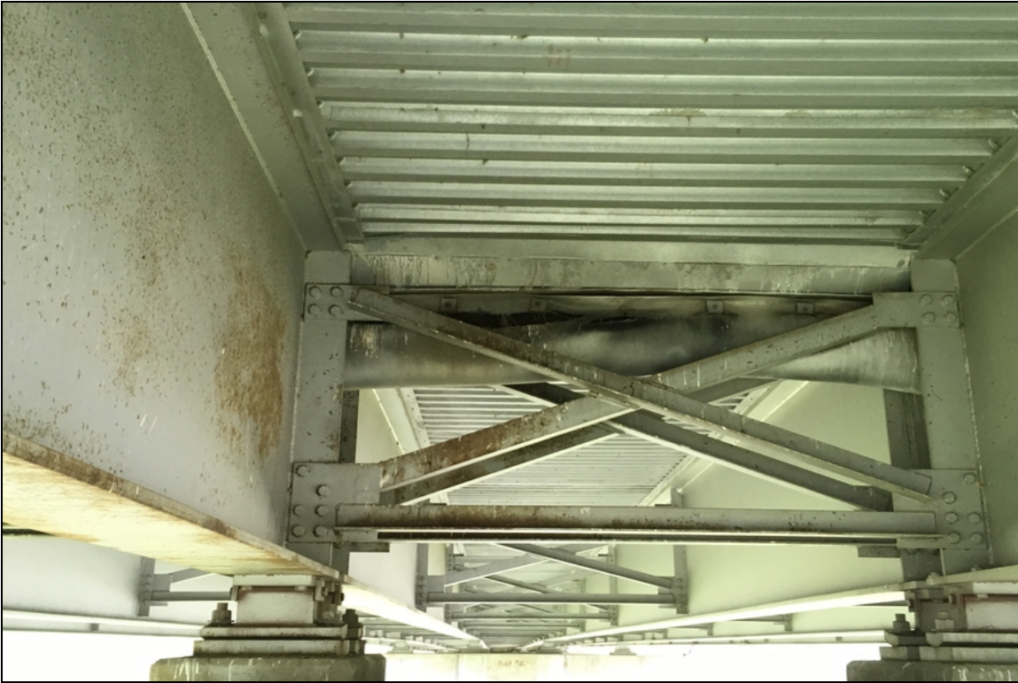
Large tear in the assembly joint trough over pier #3 on the span #4 side.
