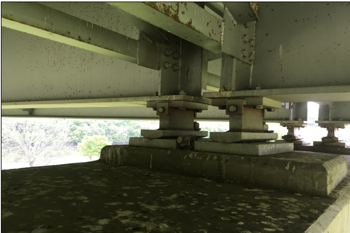
Both anchor bolts are missing on the left side of beam #5 over pier #3.
