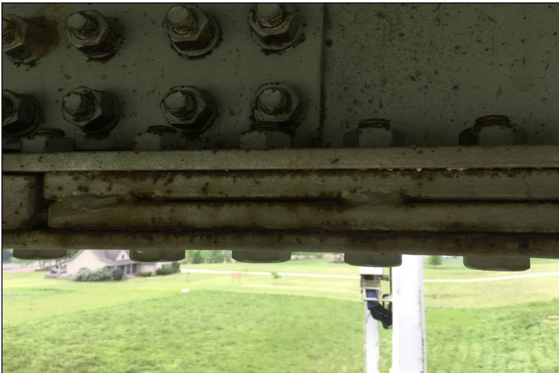
Pack rust is beginning to form on the bottom connection of the second splice in span #2.
