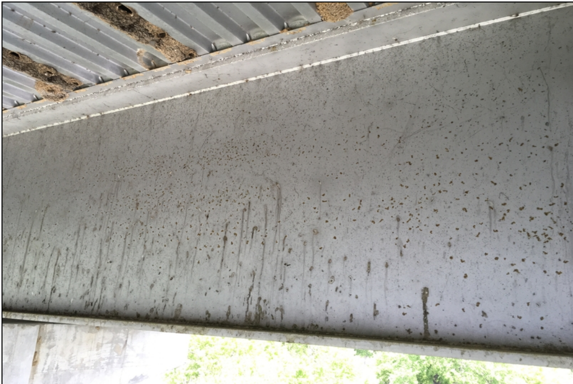
Pin point rusting in span #8 interior beams.
