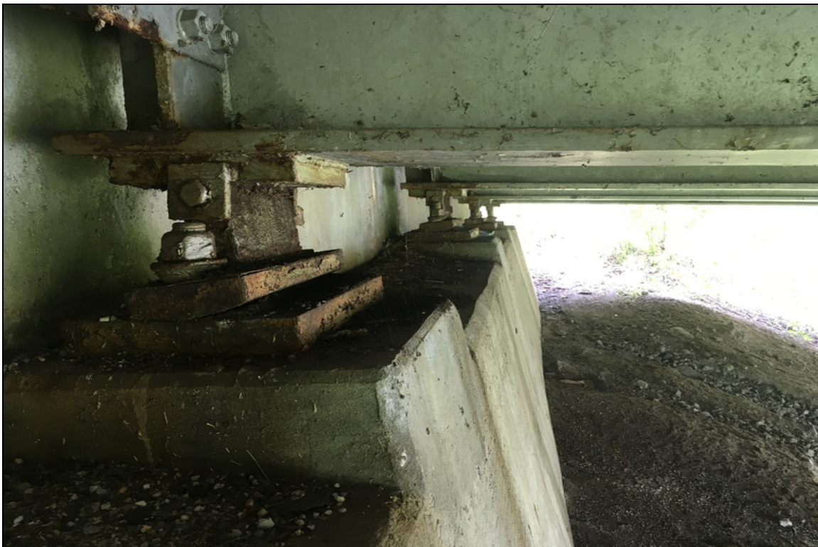
Bearings #3,4 at abutment #2. Showing tilt at 80 degrees F. The other bearings are not tilted.
