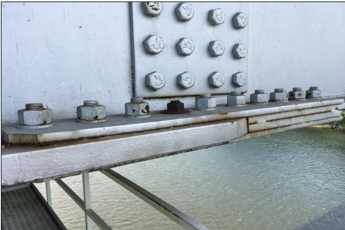
Smaller bolt in the first field splice of beam #6 in span #8. Minor pack rust has begun to form on the lower connection.
