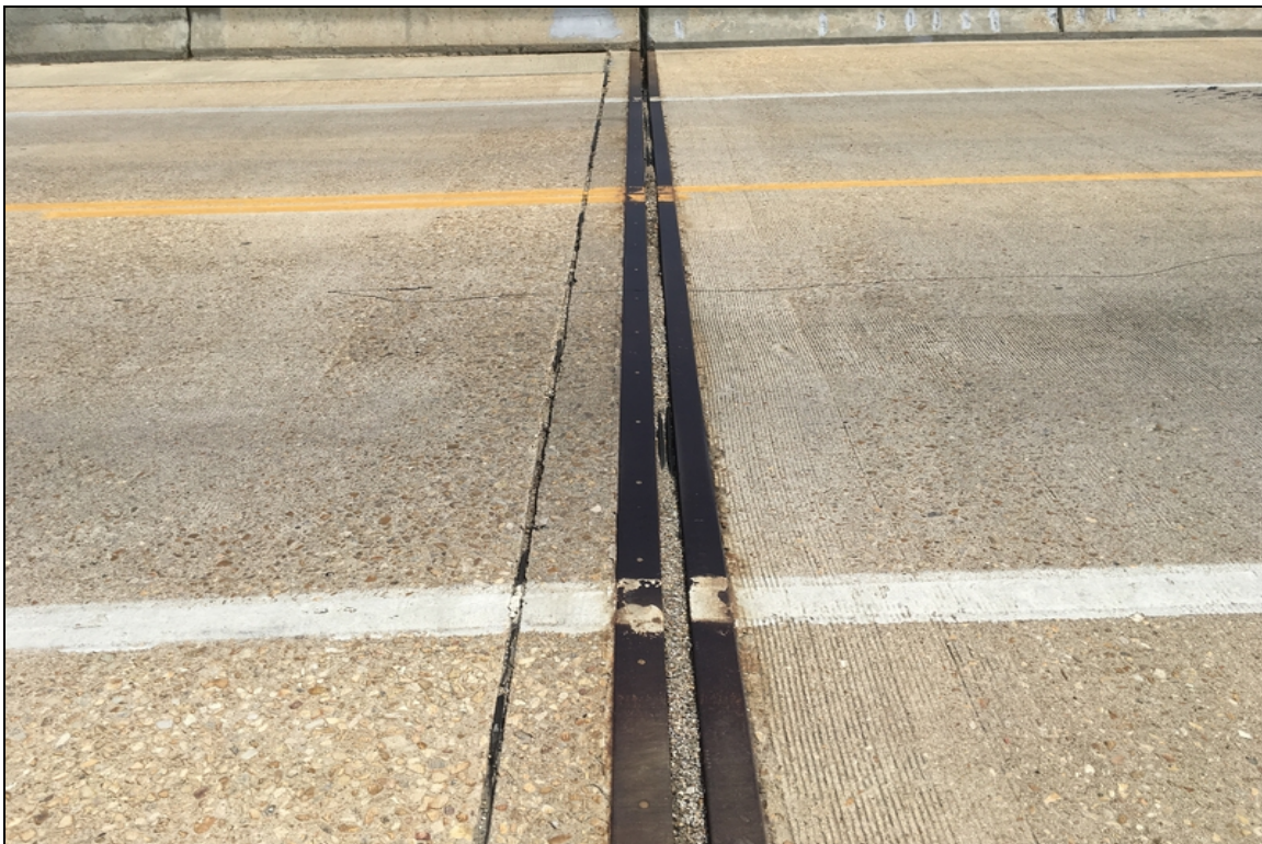
General view of the abutment #1 compression joint seal condition.
