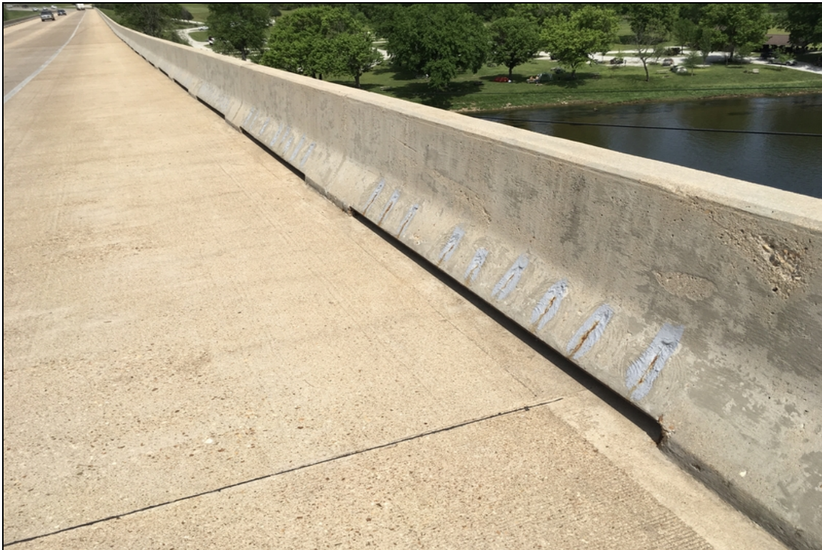
Typical view of shallow exposed rebar in the left and right parapet walls.
