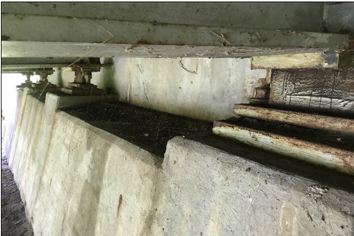
Bearing condition at abutment #2. Typical of all 6 rocker bearings at this location.
