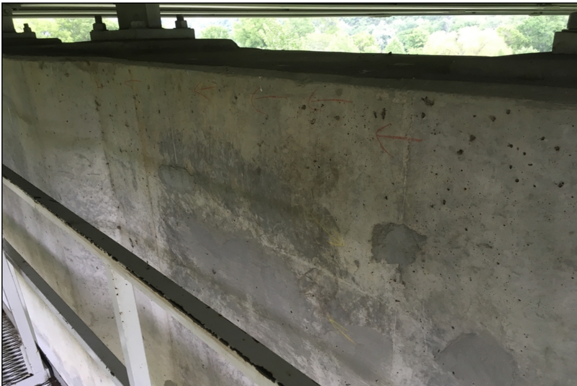
Hairline vertical Cracking in the pier caps. Typical.
