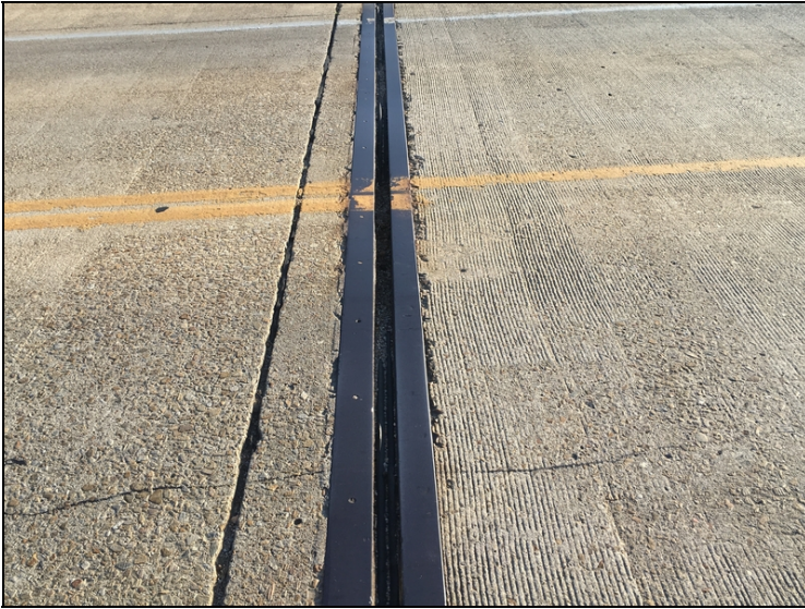
Joint seal condition at abutment 1 showing leakage and loss of adhesion.
