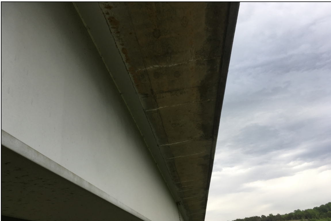
Efflorescence cracking in the left and right deck overhangs.
