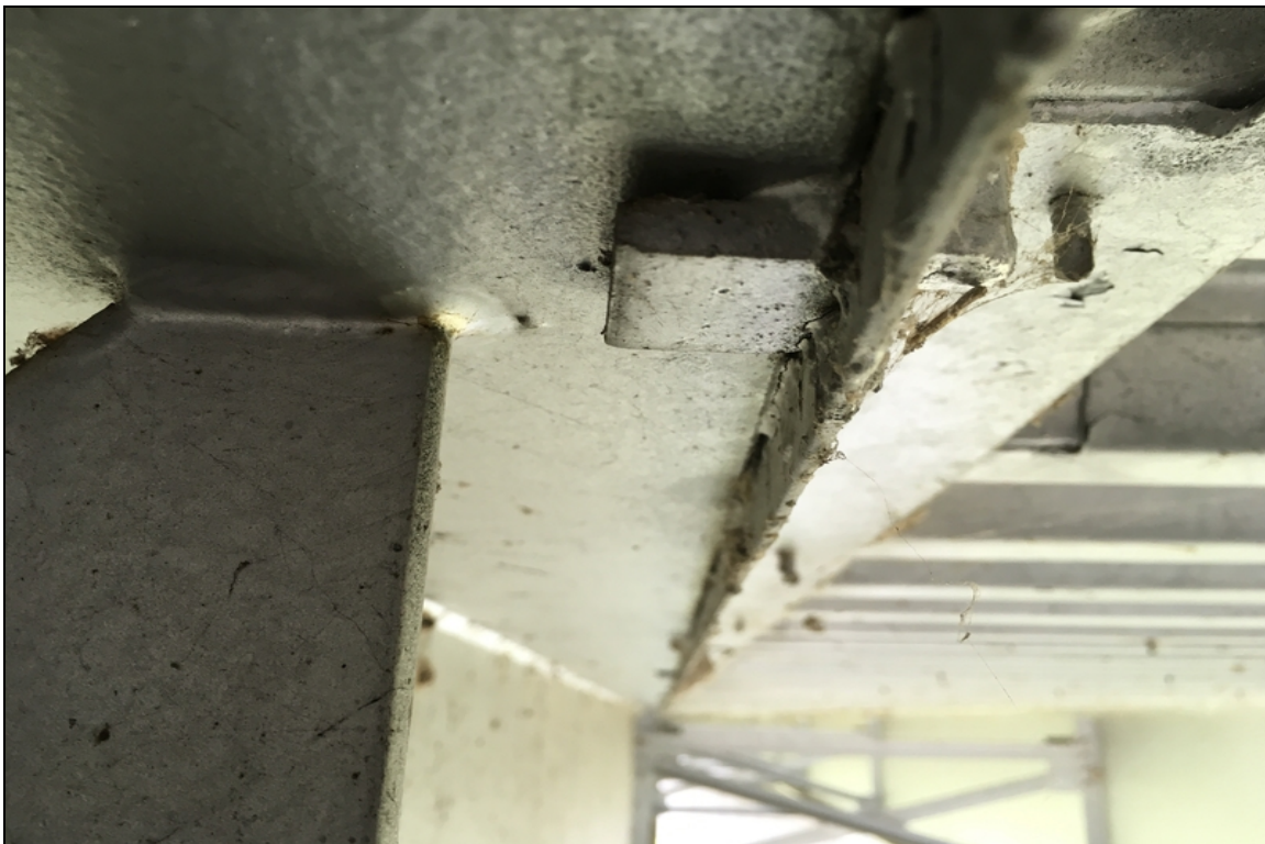
Cracked weld at upper diaphragm connection #6 at beam #6 span #6 typical of both sides of the diaphragm. Typical also of several locations in span #9 bay #5.
