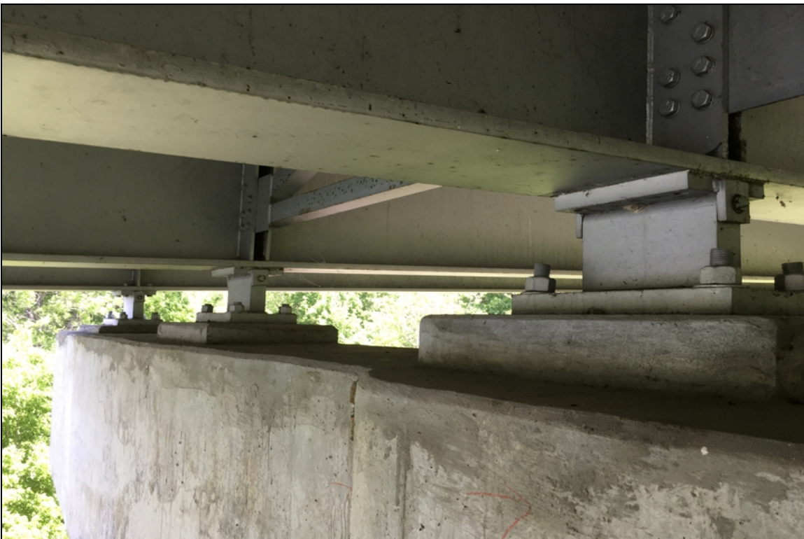
Fixed bearing condition at pier #11. Typical of all 6 at this location.
