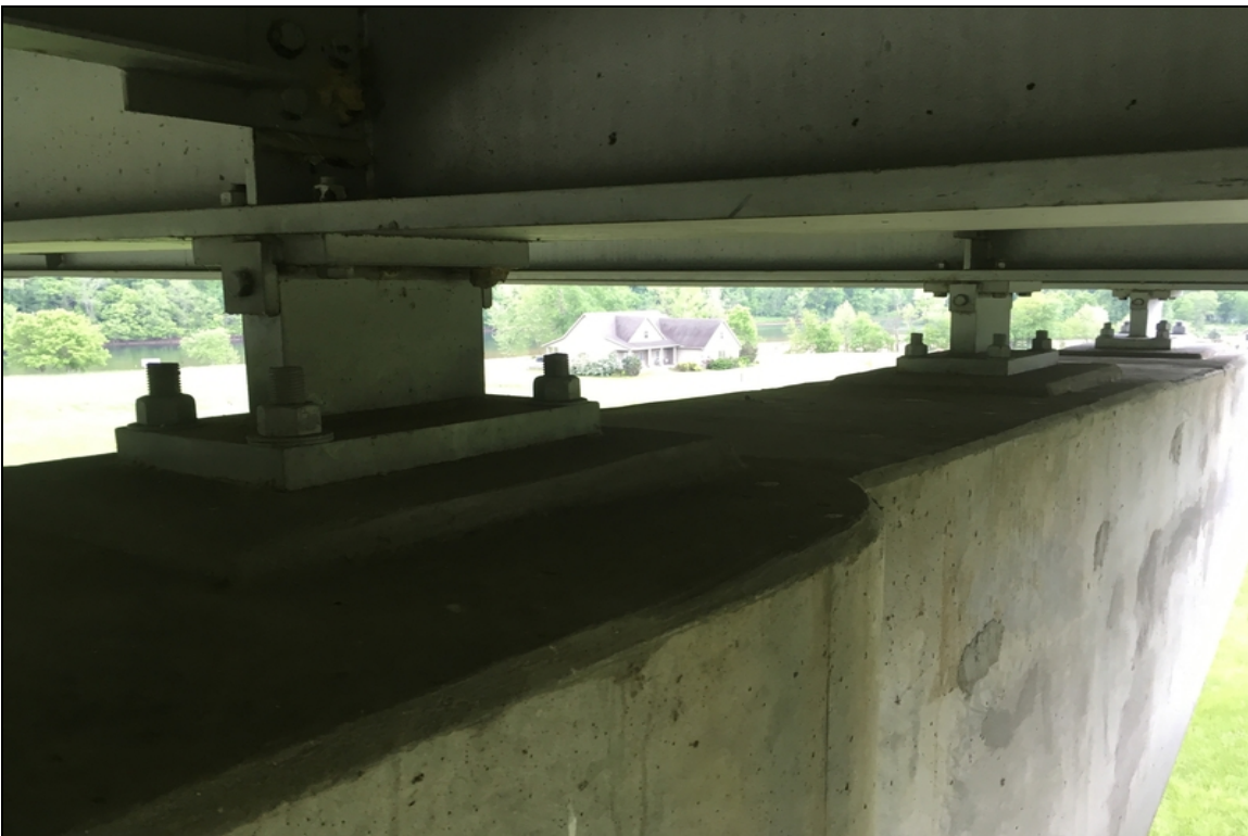
Fixed bearing condition at pier #1. Typical of all 6 at this location.
