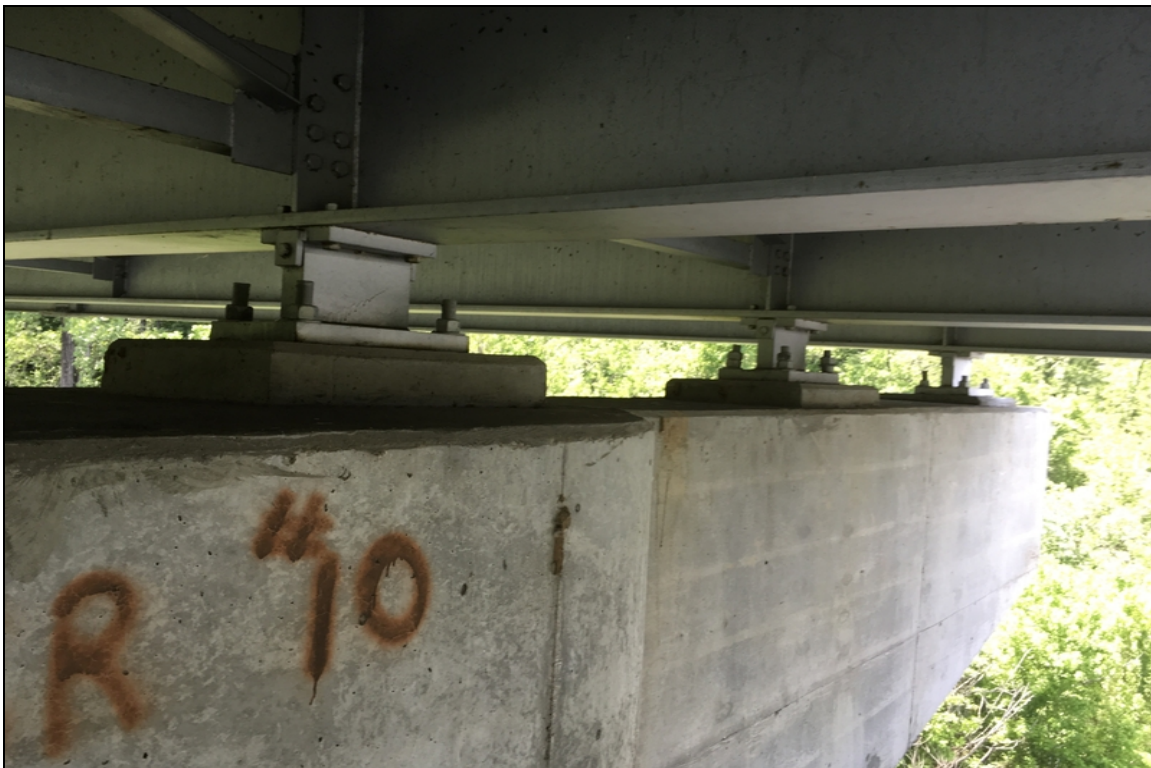
Fixed bearing condition at pier #10. Typical of all 6 at this location.
