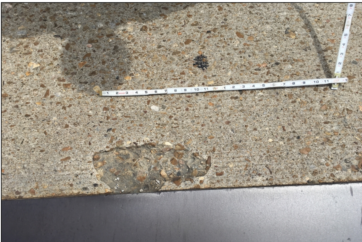
Delamination in the left driving lane at the beginning of span #4.
