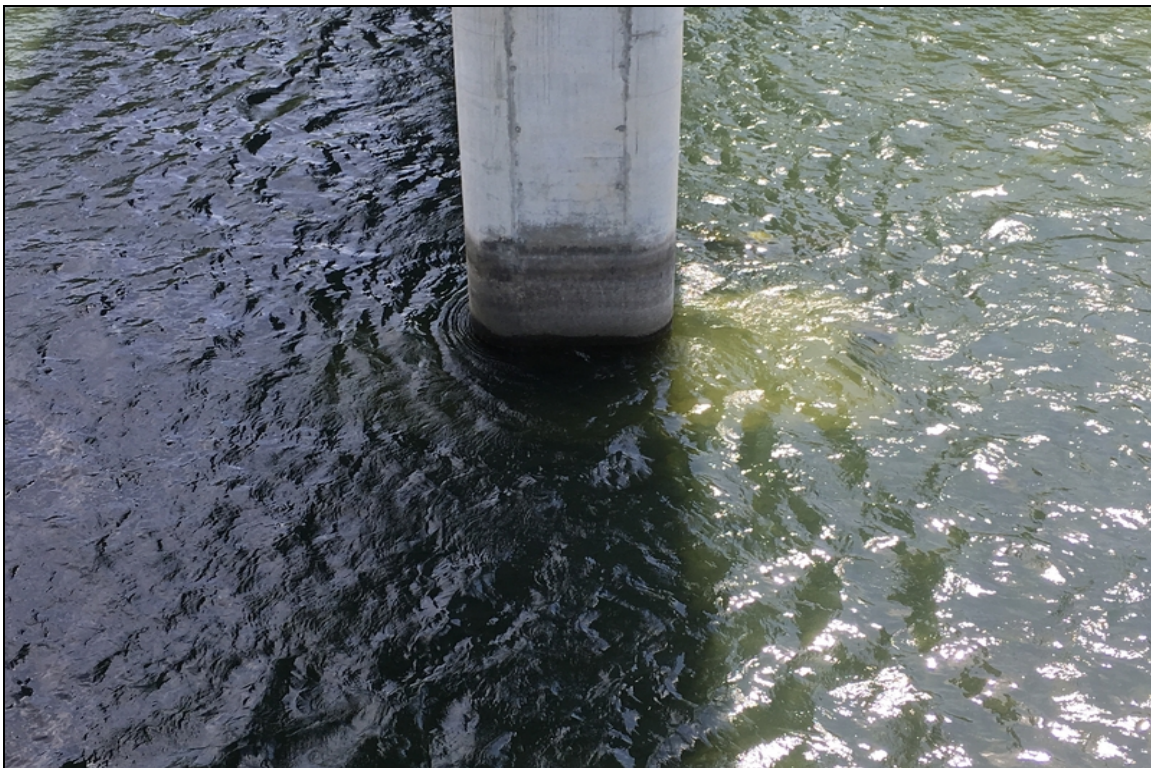
The top of the footing is fully exposed at pier #9.
