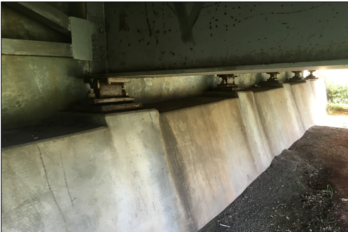
Bearing condition at abutment 1.
