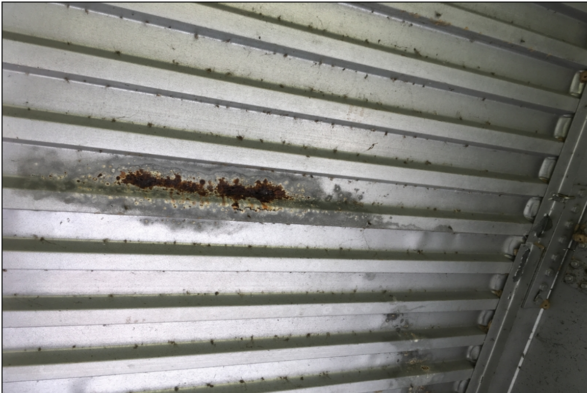
Corrosion on the sip forms in span #7. Typical of several bays in several spans.
