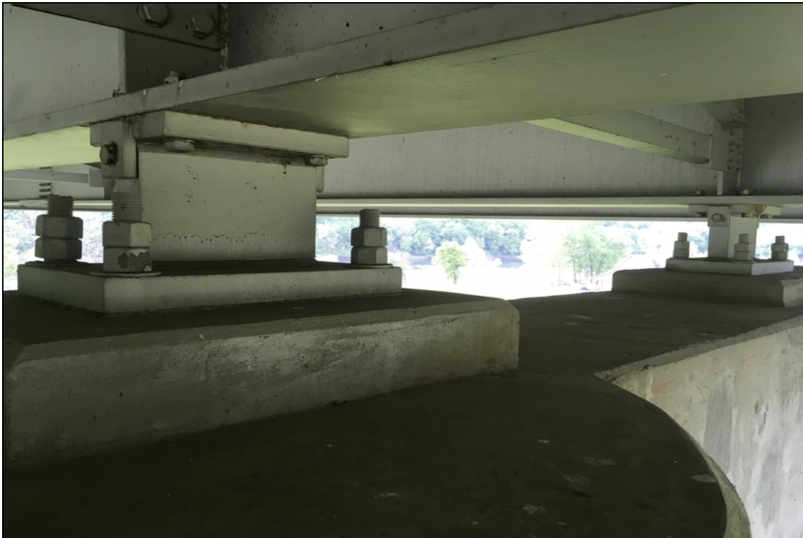
Pier #2 bearing condition. Typical of all 6 at this location.
