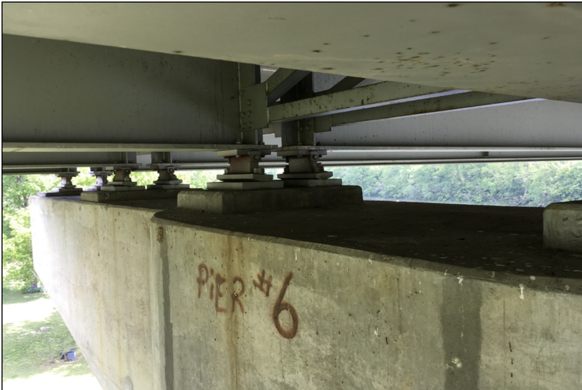
Moveable bearing condition at pier #6. Minor corrosion with no section loss. Typical of all 12 at this location.
