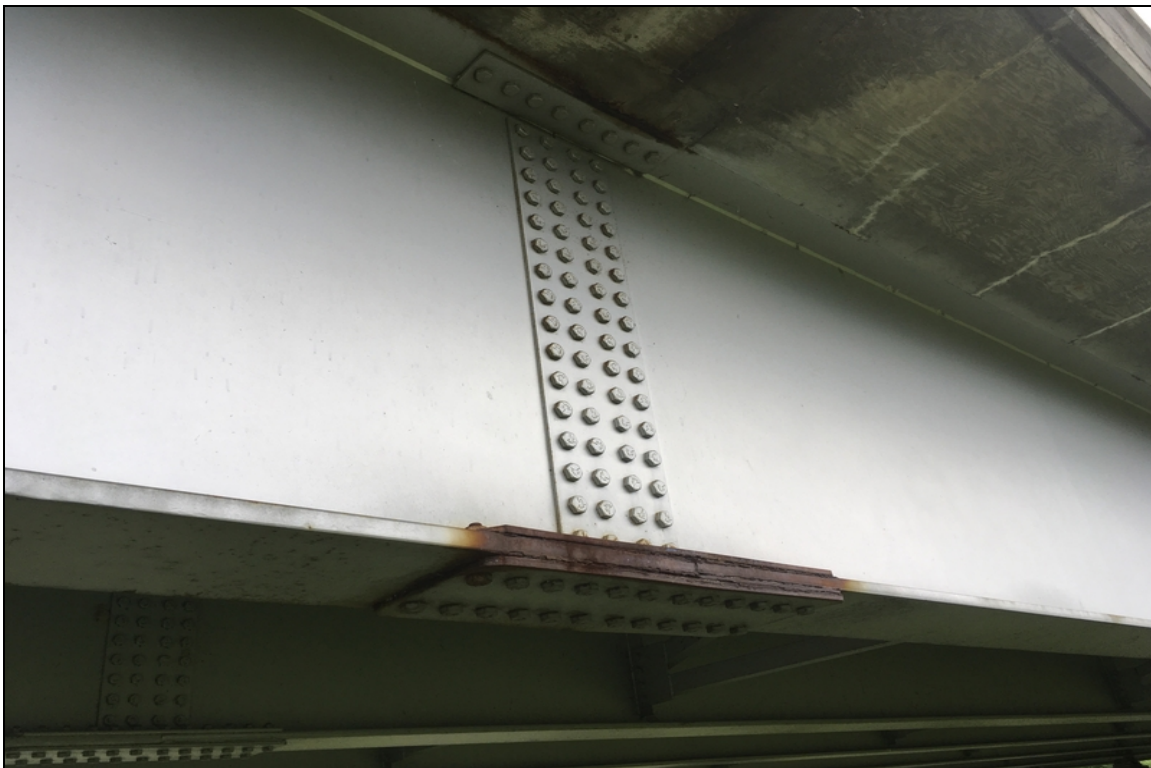
Corrosion with pack rust on the splice panel of beam #6 span #3.
