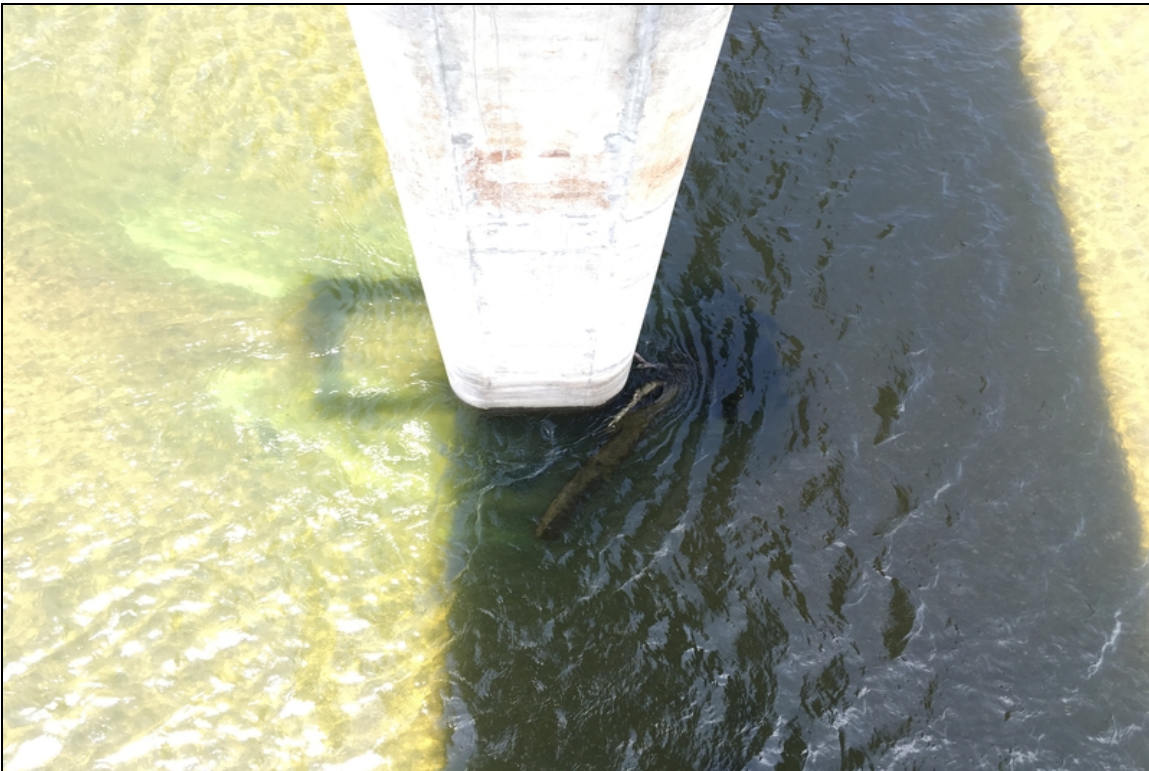
Minor drift accumulation on pier #8.
