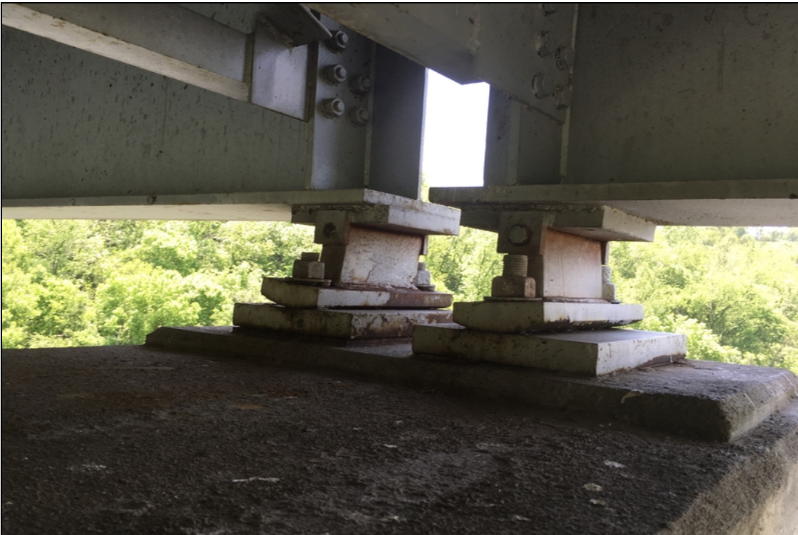
Exterior bearing condition at pier #9. Typical of the 4 outside bearings. Note the sheared sole plate connection bolt at beam #6. The sole plate bolt is missing on both sides of the bearing.
