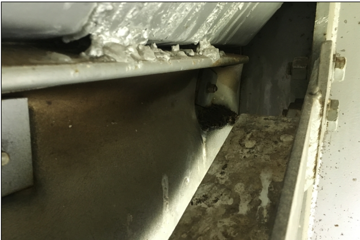
Torn location on the neoprene trough in bay #2 over pier #3.
