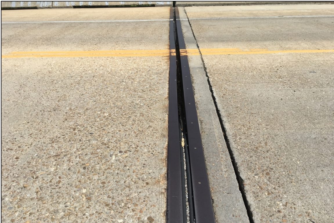
General view of the abutment #2 compression seal.
