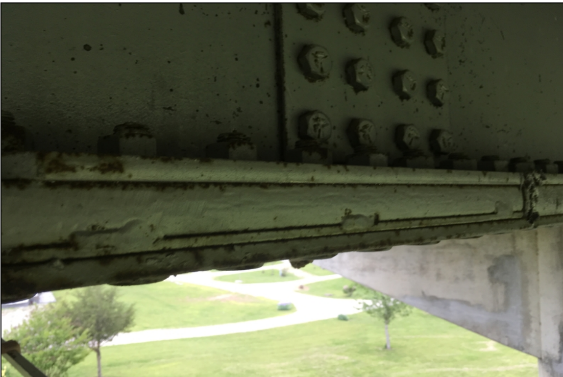
Tack welds on the spacer plates of the splice panels. Typical of all locations.
