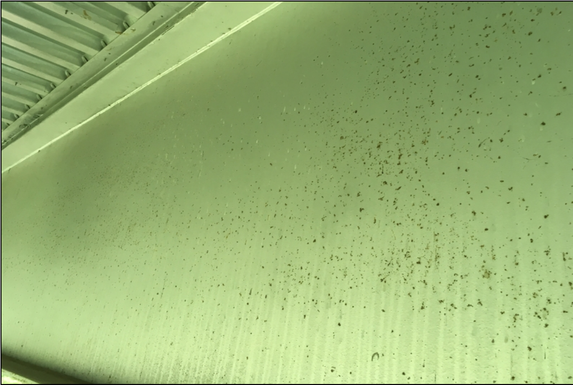
Pin point rusting on beam #4. Worst case condition in span #2.
