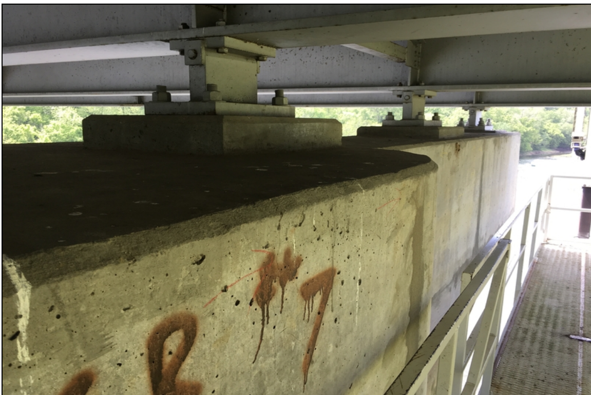
Fixed bearing condition at pier #7. Typical of all 6 at this location.
