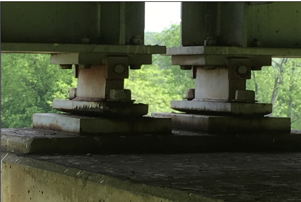
Bearing condition at pier #3 under girder #1. Showing corrosion at the rocker area.
