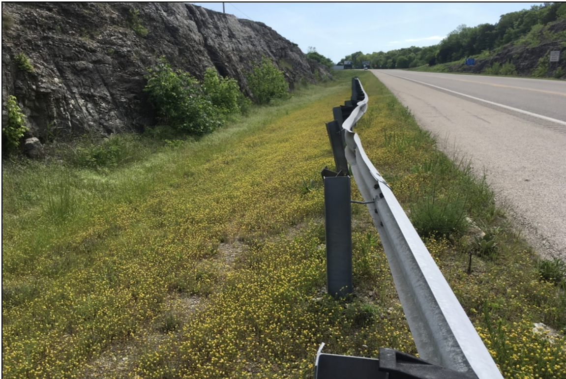
The left ending approach railing has 26' of vehicle damage.
