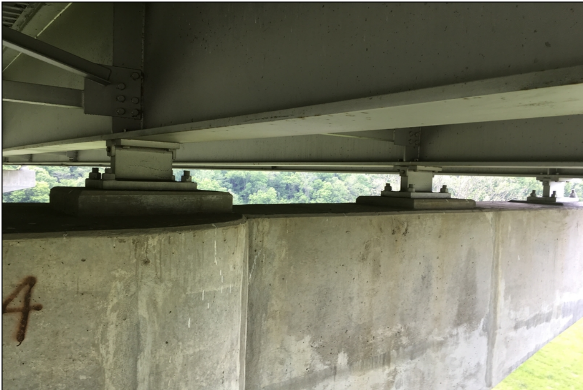
Fixed bearing condition at pier #4. Typical of all 6 at this location.
