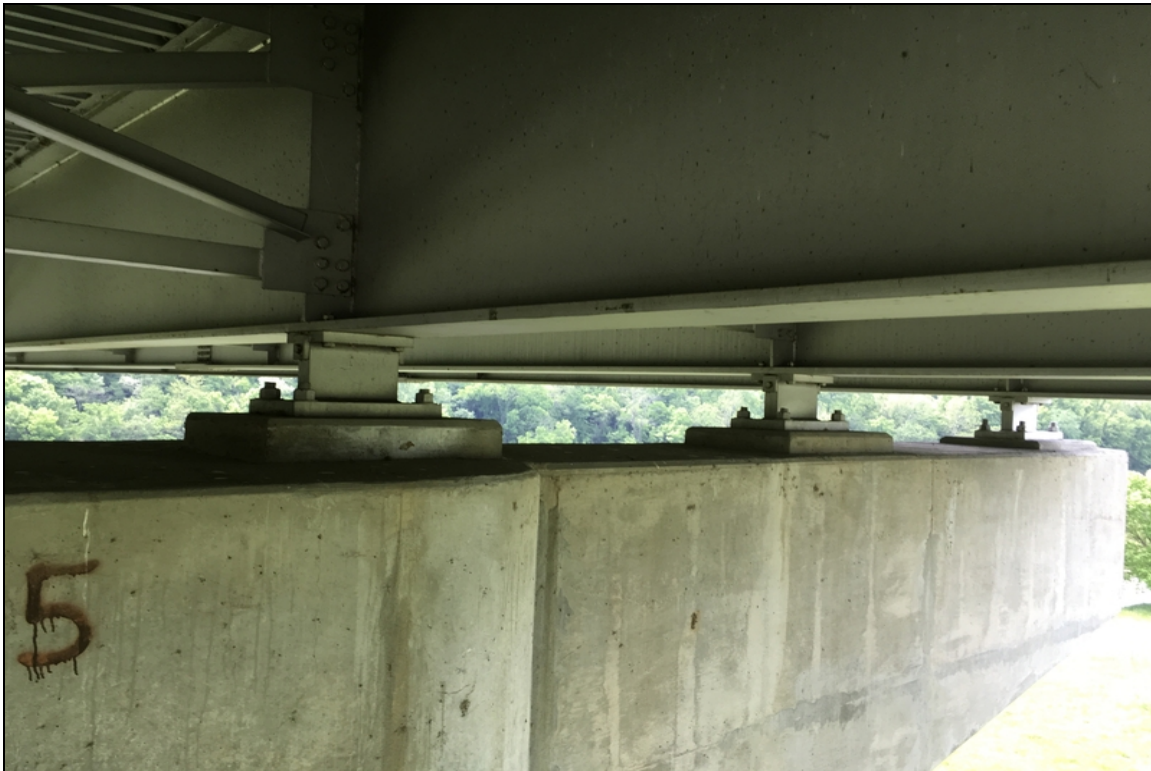
Fixed bearing condition at pier #5. Typical of all 6 at this location.
