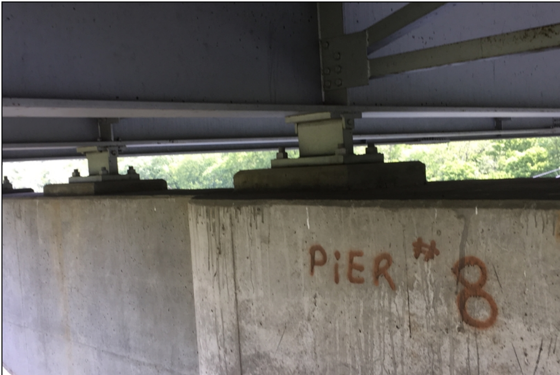
Fixed bearing condition at pier #8. Typical of all 6 at this location.
