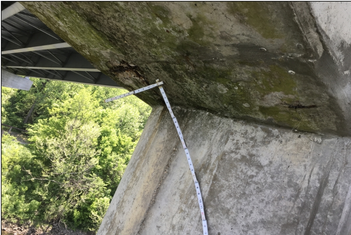
Spall with exposed rebar on the underside of the left cantilever of pier #9.
