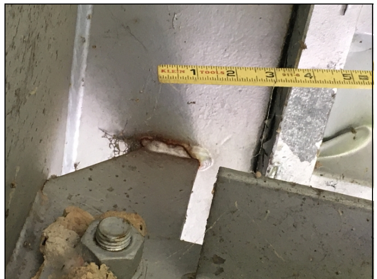
Fully cracked upper diaphragm weld on diaphragm 4 on beam 6 in span 11.
