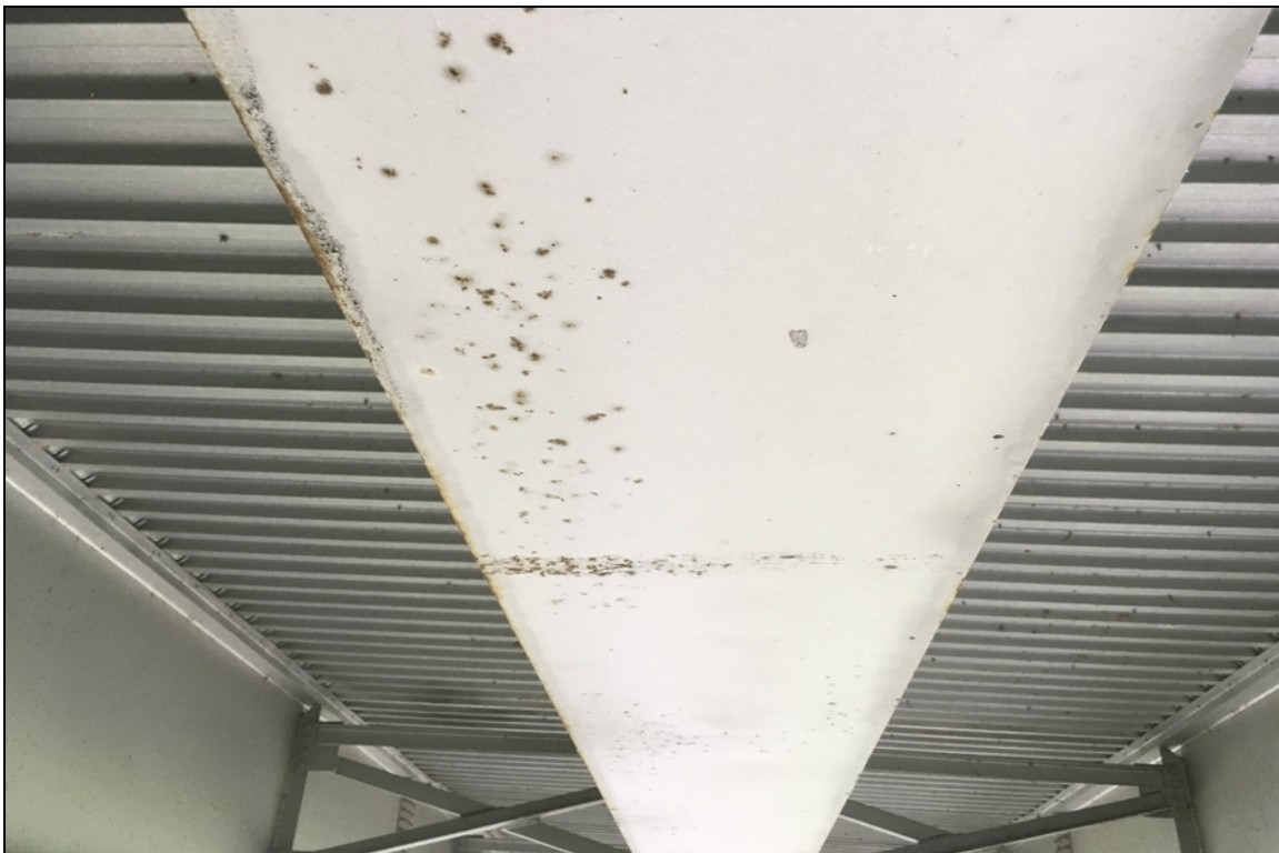
Typical paint condition of the bottom flanges of all beams.
