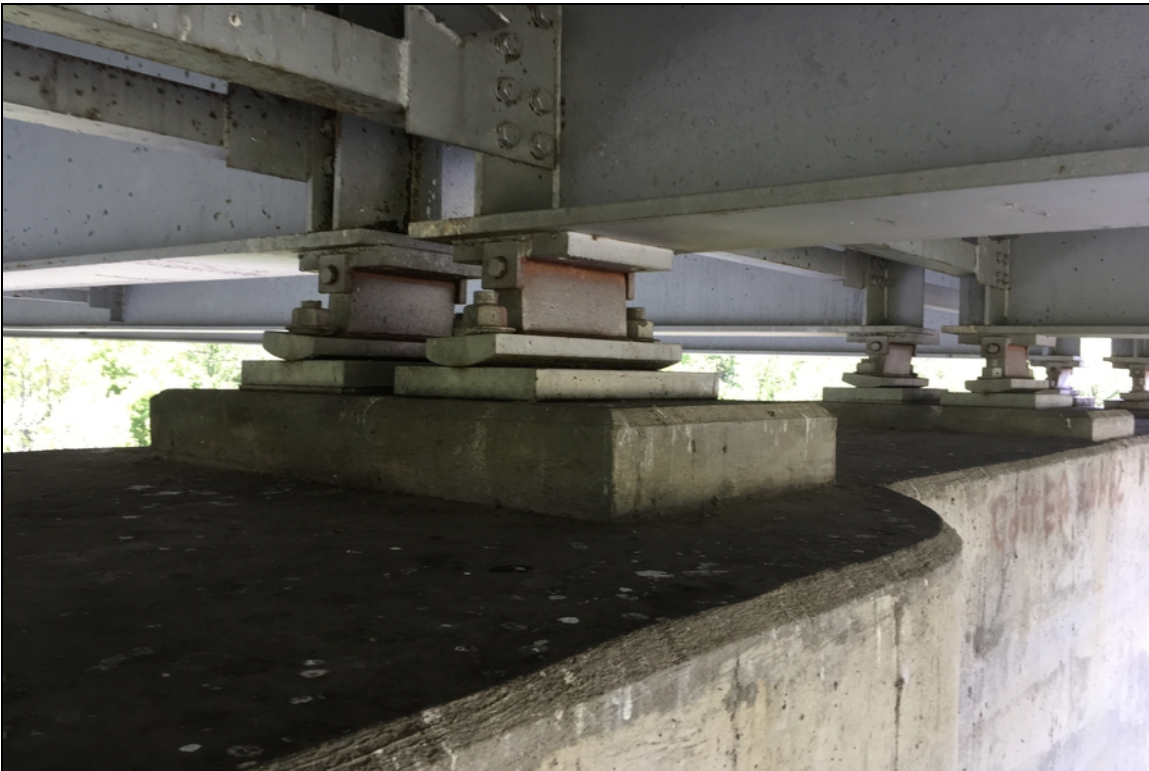
Moveable bearing condition at pier #9. Typical of the 8 interior bearings.
