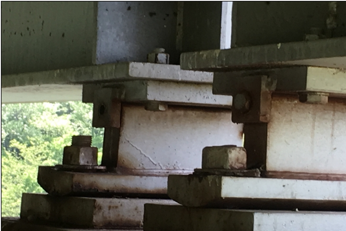
Moveable bearing at pier #6 girder #6 has a missing sole plate connection bolt.
