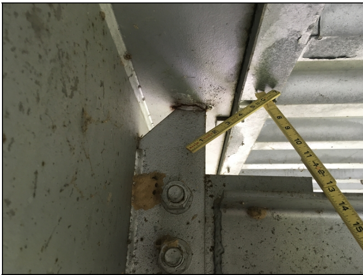
Fully cracked weld in the top of diaphragm 4 in span 5 on beam 6.
