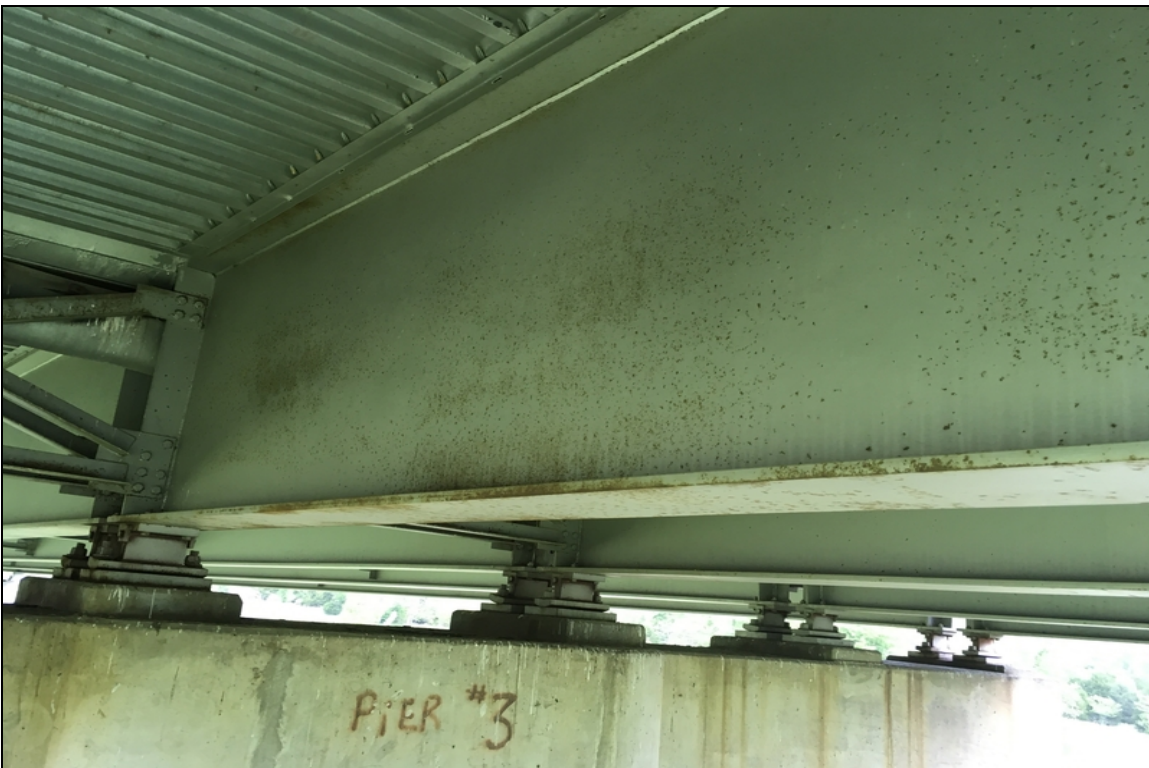
Minor corrosion for 20' on beam #4 in span #4.
