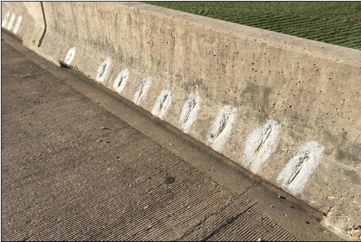
Exposed rebar in the concrete parapet walls.
