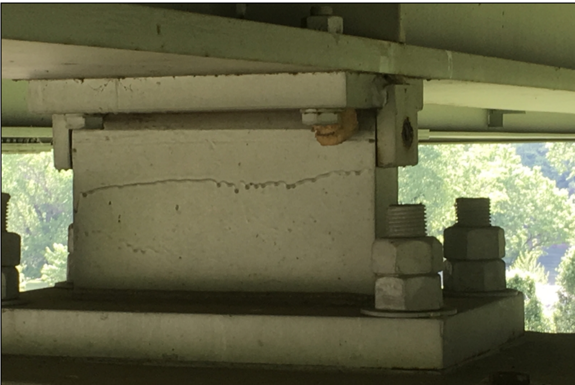
Sole plate bolt is missing on the right side of girder #3 at pier #2.
