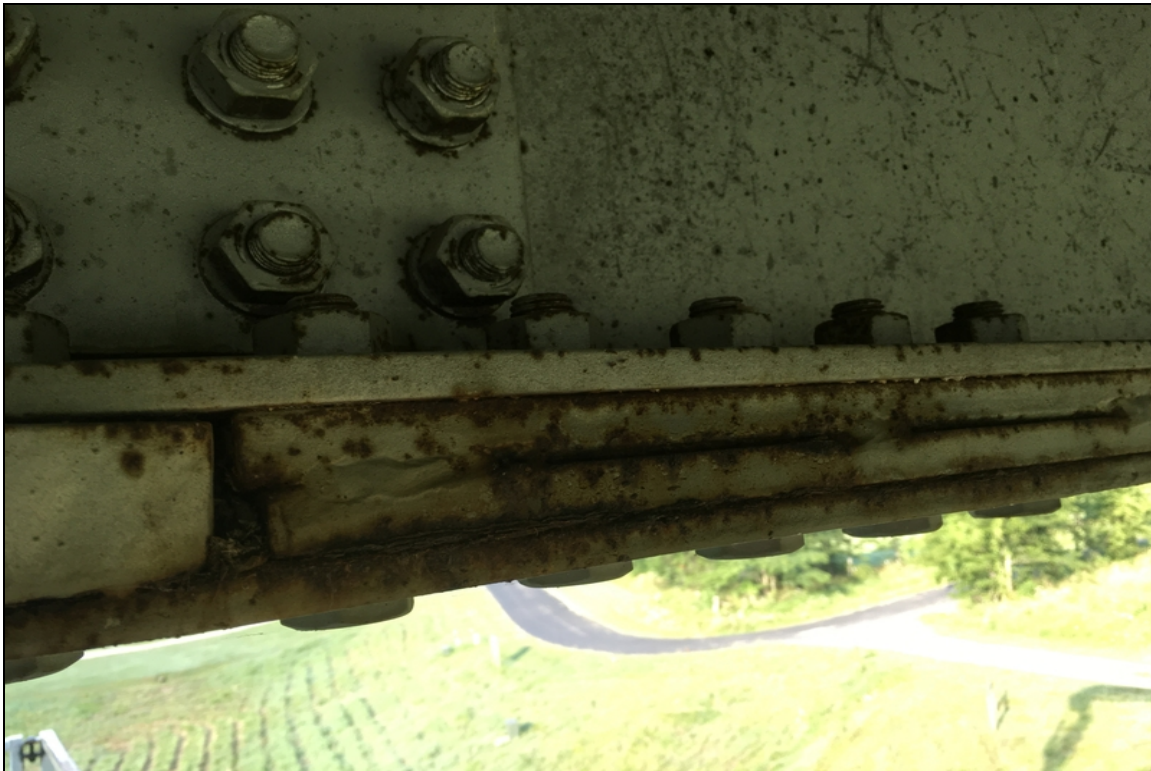
Pack rust is beginning to form at splice panel 2 on beam 6 in span 2
