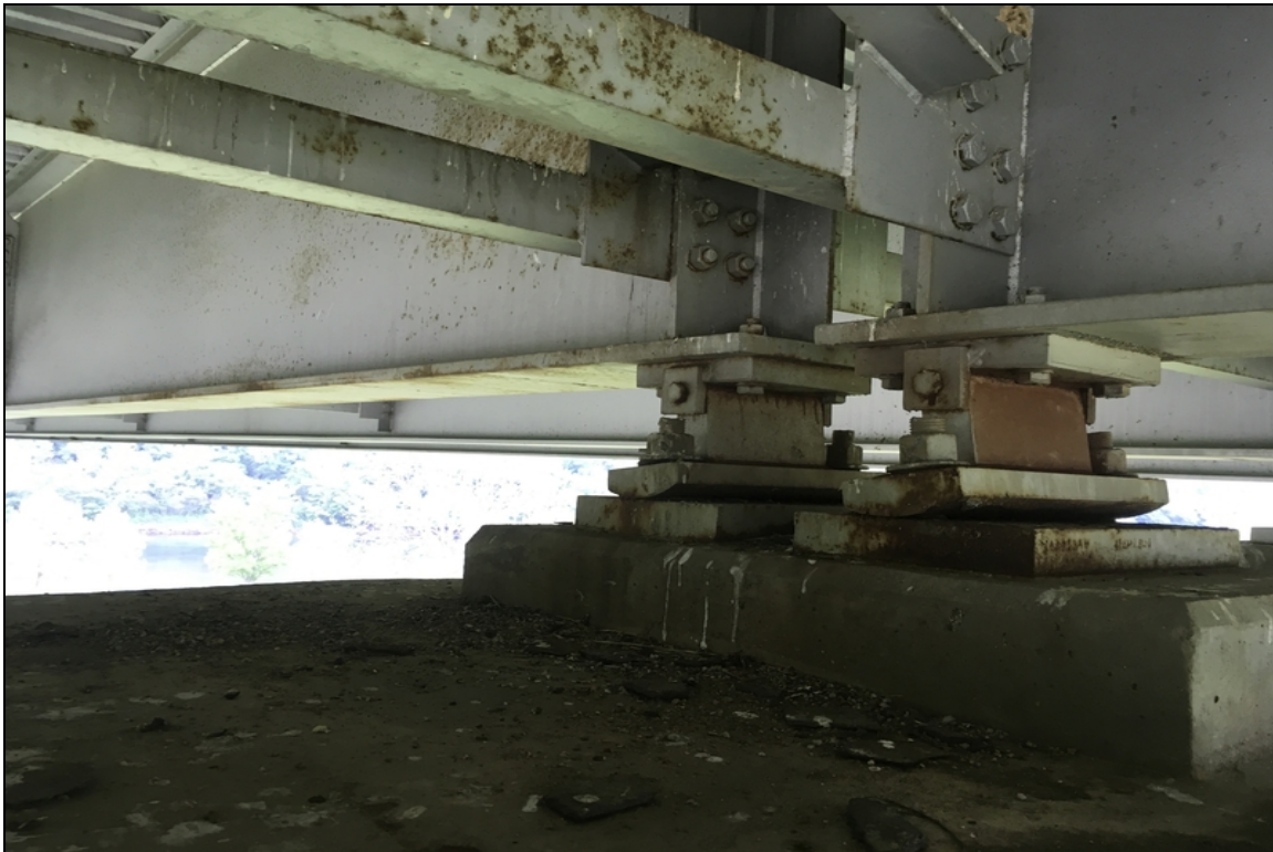
Condition of the 8 interior moveable bearings at pier #3.
