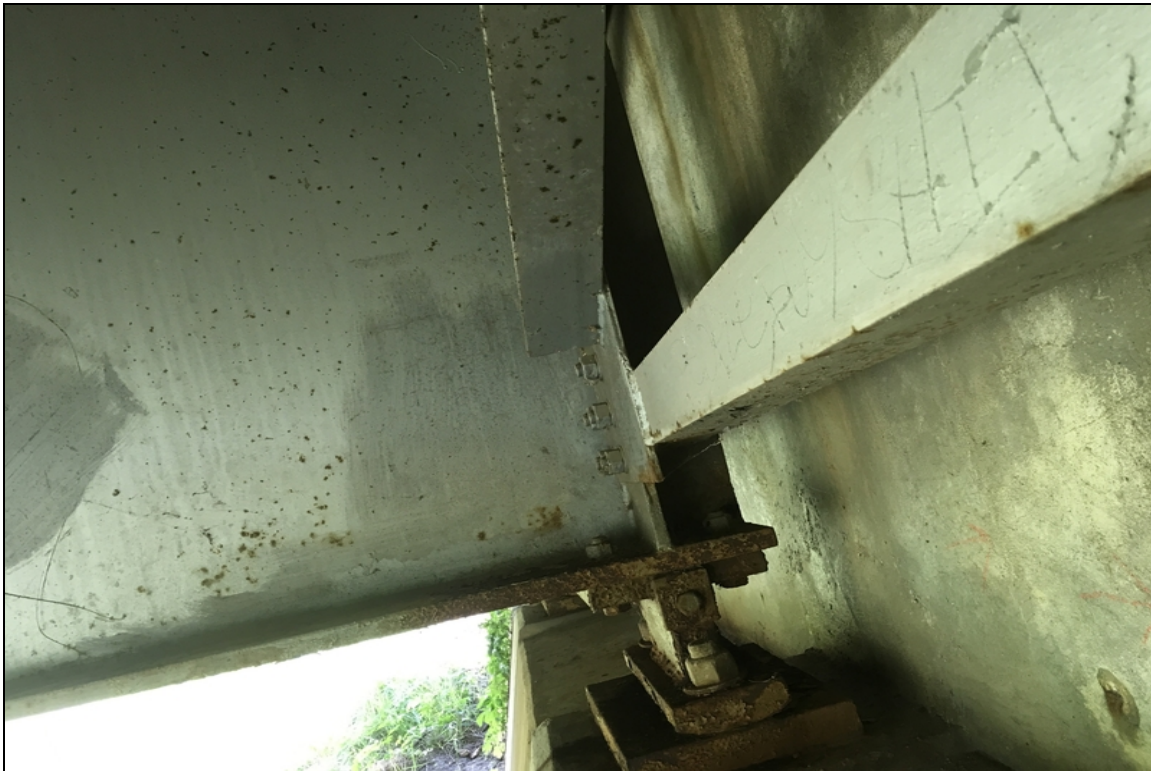
Beam end corrosion at abutment #1 due to leaking joint seals.
