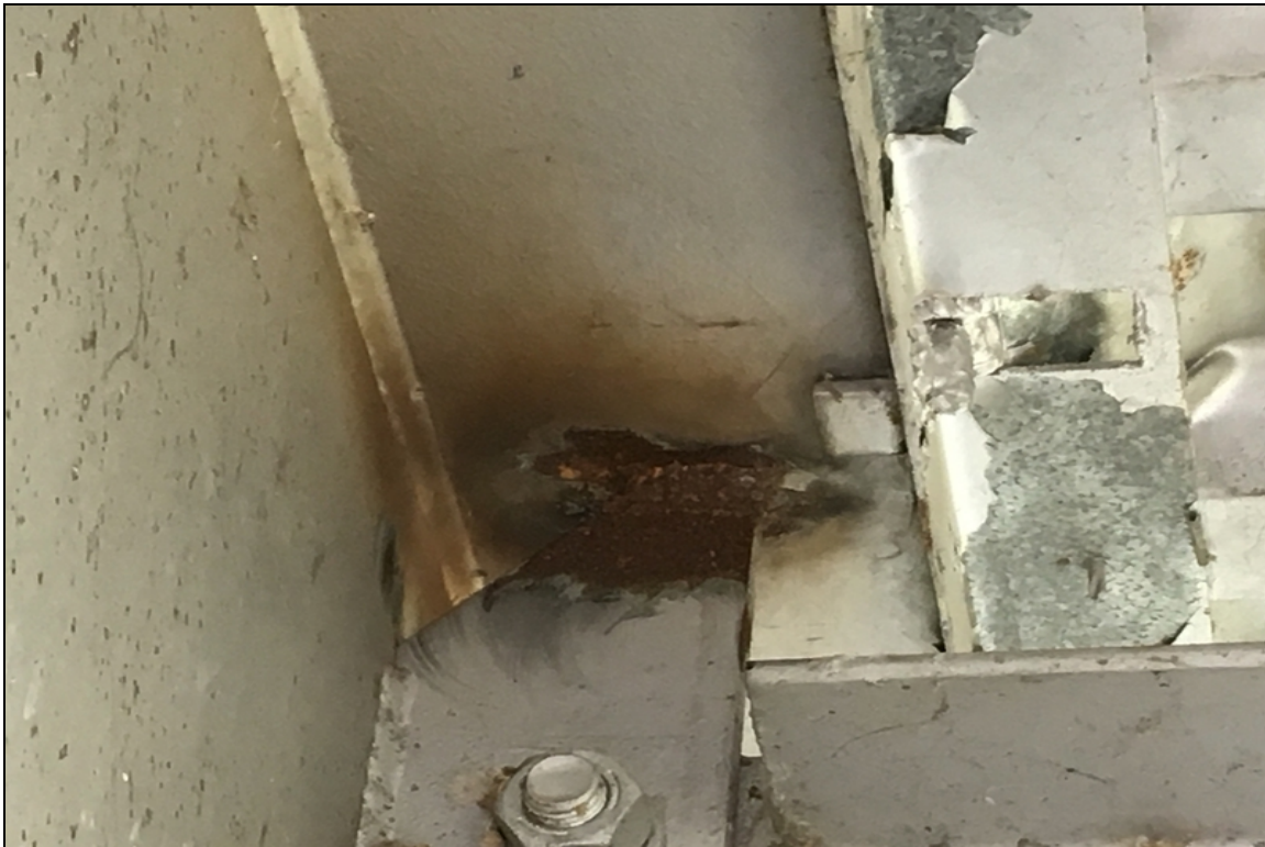
Re welded upper diaphragm connection on girder #6 of span #6 near mid span.
