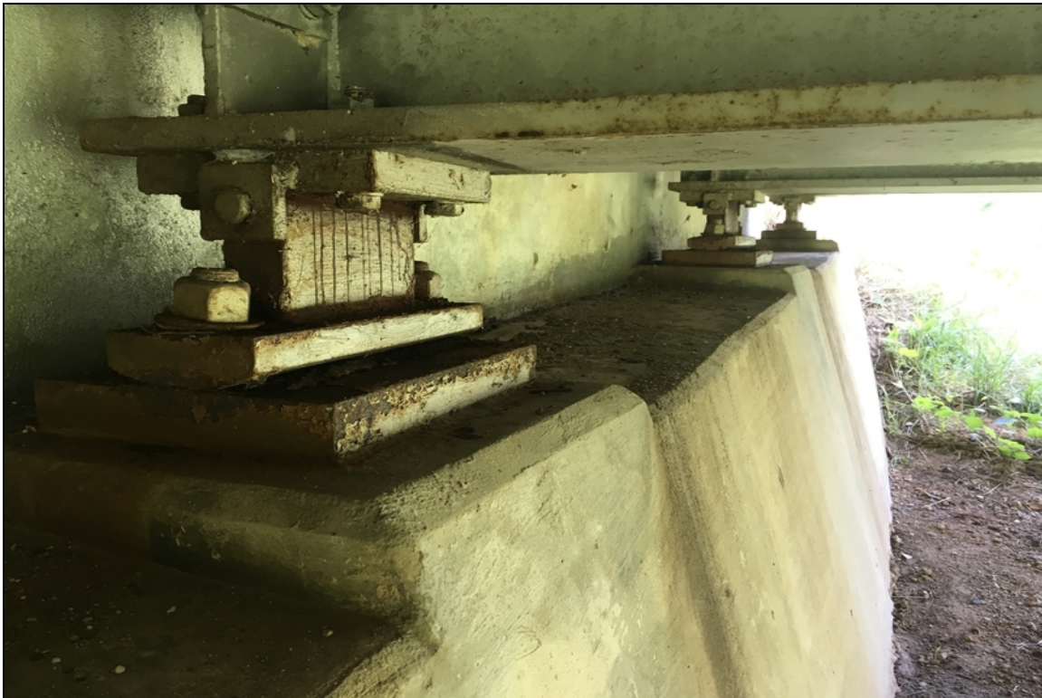
General view of abutment #1 moveable bearings. Typical of all 6 at this location.
