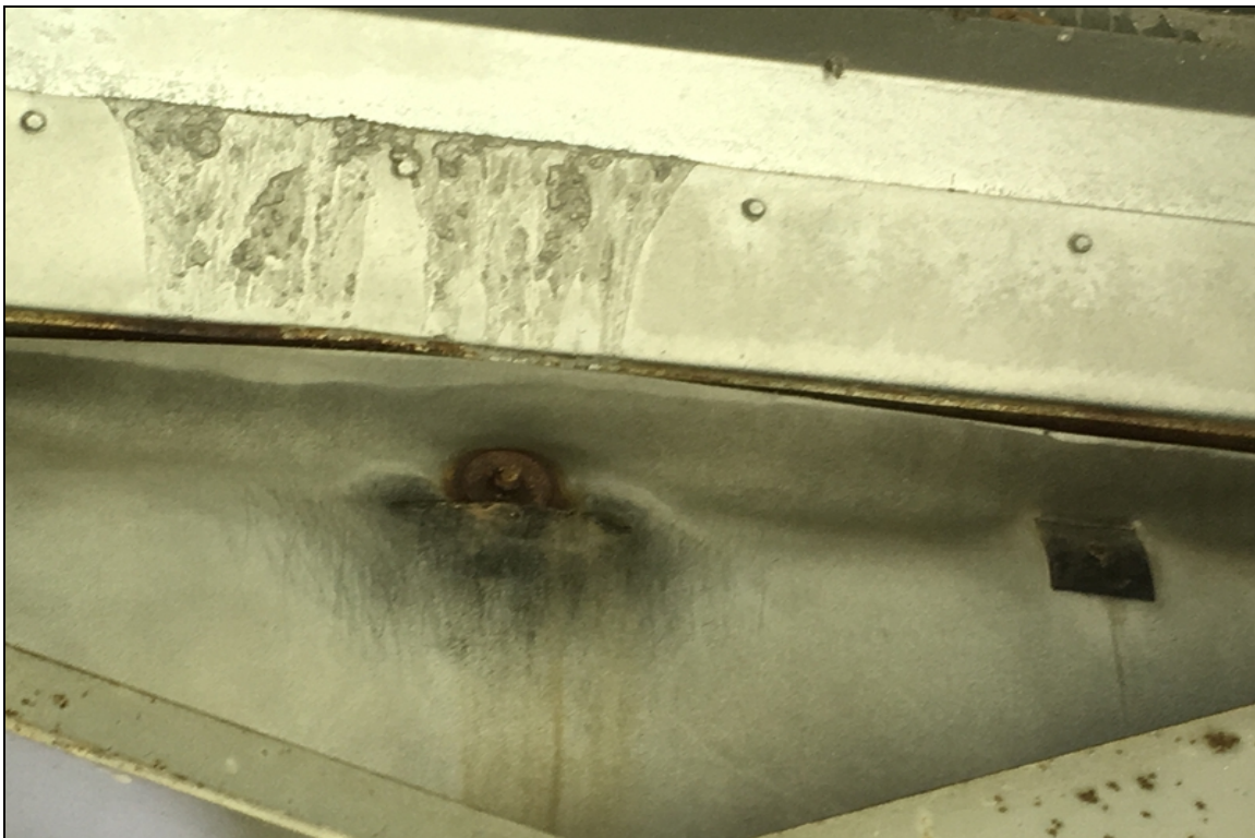
Tears in the trough connections at the pier #6 assembly joint.
